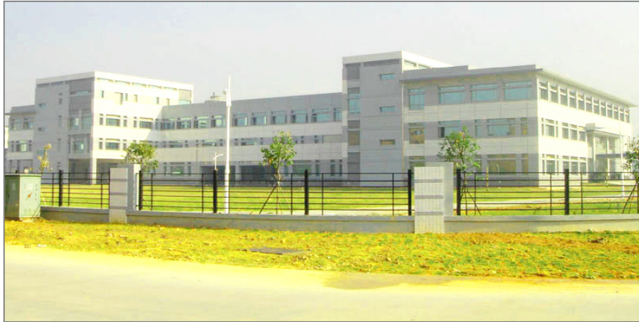
EG-Billion New Plant at Shijie, Dongguan China
